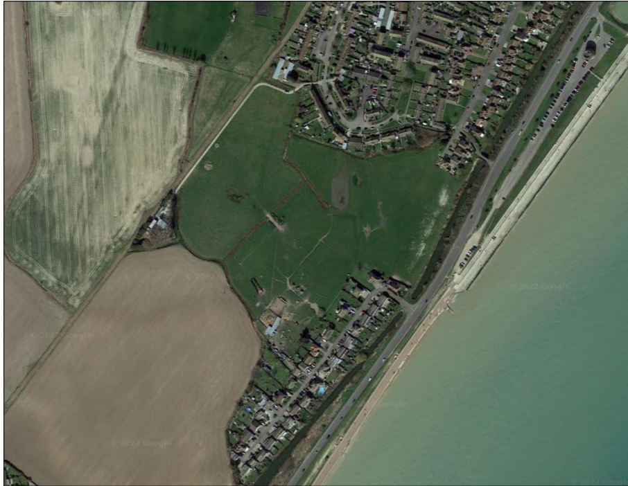
Fig.1: Aerial photo centred on site (dark green)
